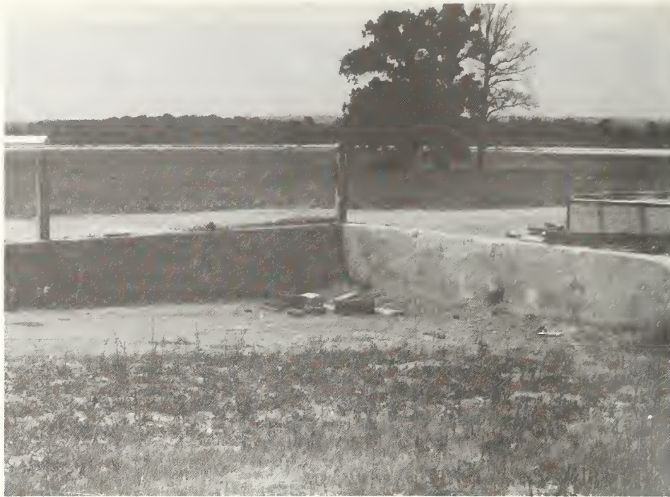
Loading Dock Overall View
